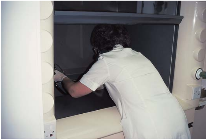
Fig. 6.1 Fume cupboard in endoscopy unit – designed so that nurses have to put their heads inside in order to wash endoscopes!
