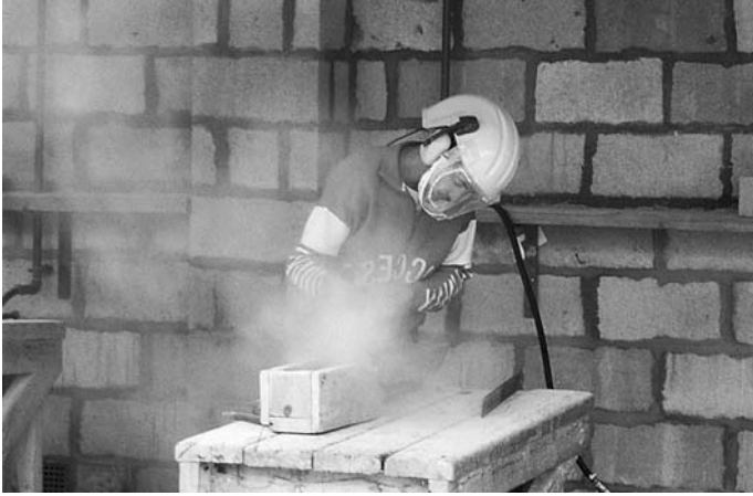
Fig. 3.1 Stonemason generating cloud of quartz dust in cutting sandstone. See also colour plate 3.1.
