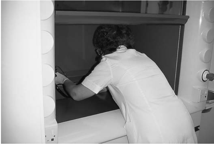
Fig. 6.1 Fume cupboard in endoscopy unit – designed so that nurses have to put their heads inside in order to wash endoscopes! See also colour plate 6.1.
